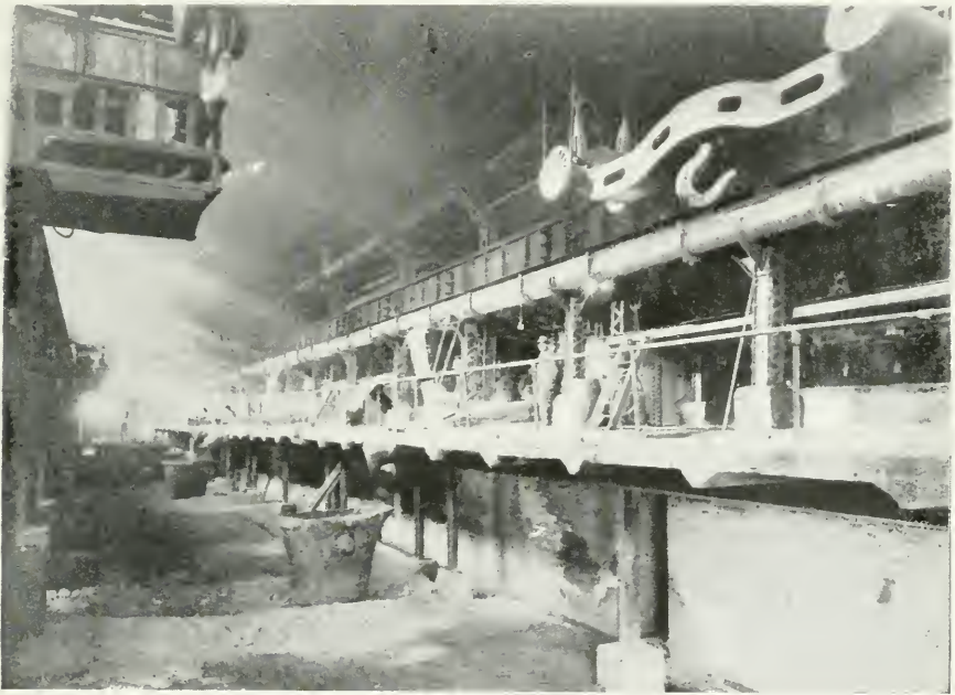
Fig. 70—Blast Furnace Tapping Floor, Copper Cliff.
